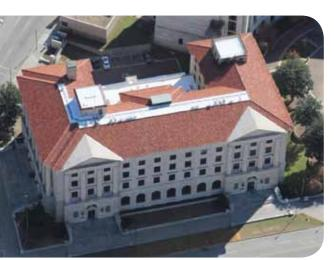
ply membrane. The self-adhering base sheet allowed an easier installation and the SRI on the cap sheet was as high and higher then some single plys. This asphalt system is aesthetically-pleasing, waterproof and includes the specifications to meet energy codes and historic codes without sacrificing quality.
