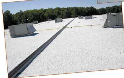
Above: The State Capitol building in Frankfort, Kentucky was re-roofed using a 2-ply modified bitumen roofing system from Siplast, an ARMA member. The base layer of modified bitumen was installed in hot asphalt and the modified cap sheet was installed with cold process adhesive. (Photo courtesy of Patrick D. Murphy Co., Inc.)
